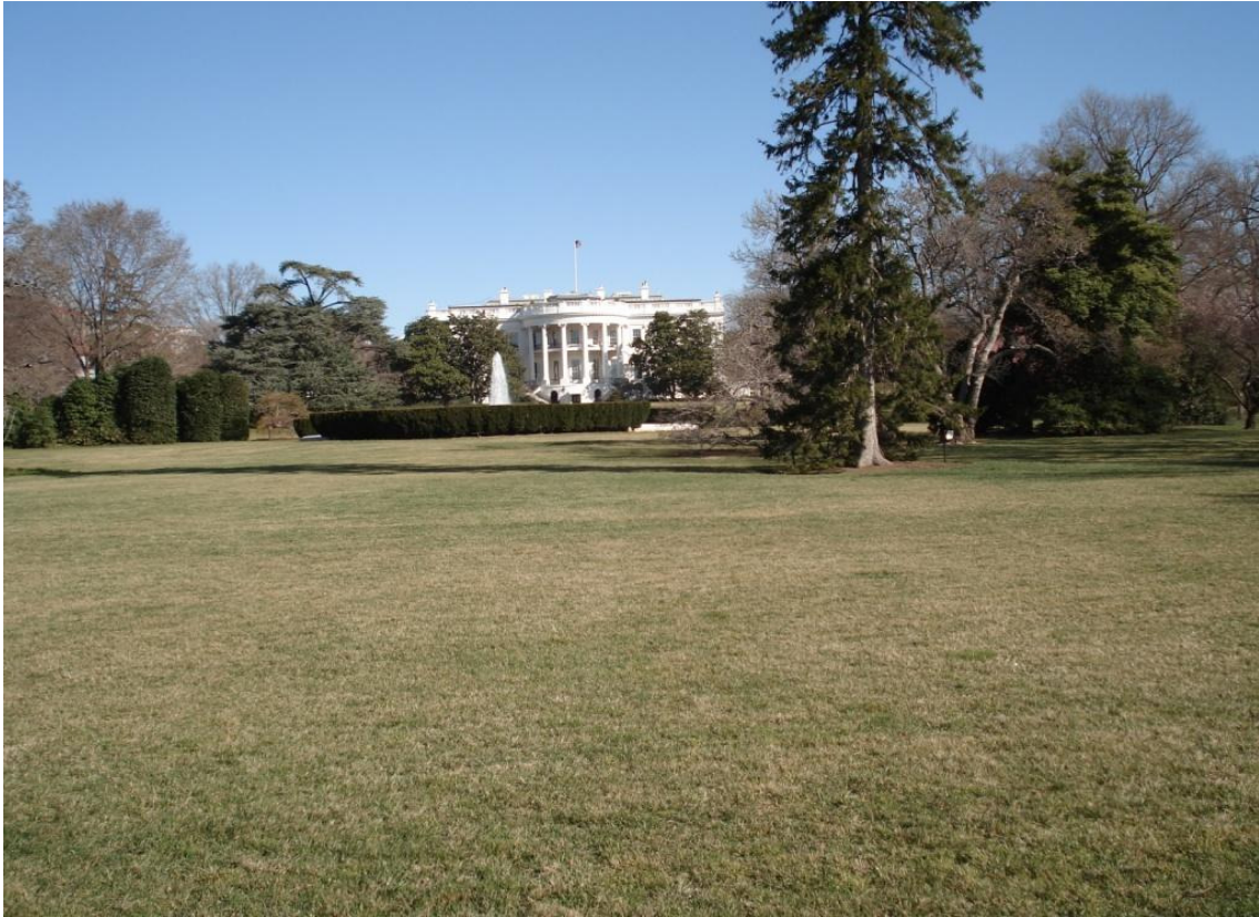
The White House seen from the Southside on 9 th March 2009
